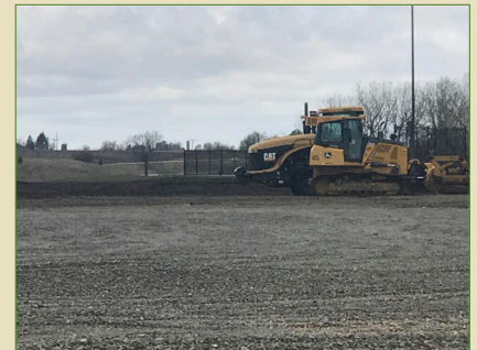
Dirt work for new fields!
