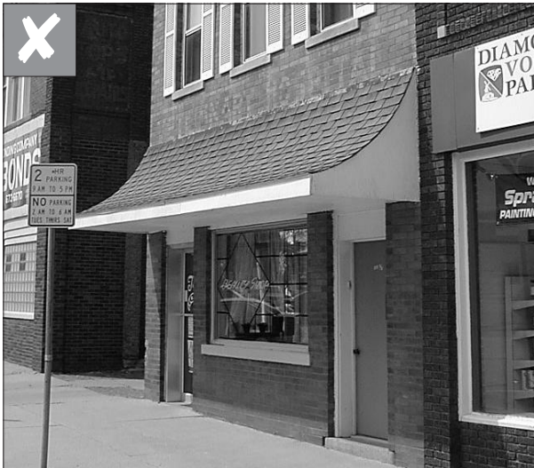
A rigid awning or canopy that is permanently attached to the building front and out of character of the building style is inappropriate.
