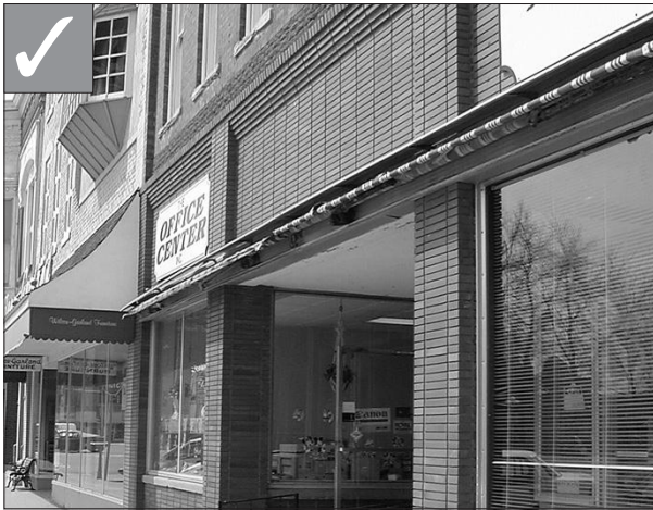
Operable awnings are encouraged on historic buildings.
