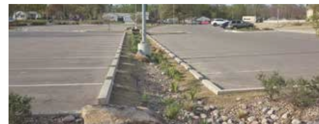
A bioswale example of how parking lots can be design to manage stormwater and water quality
