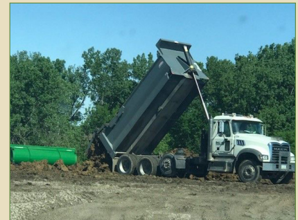
Work continues for new fields!
